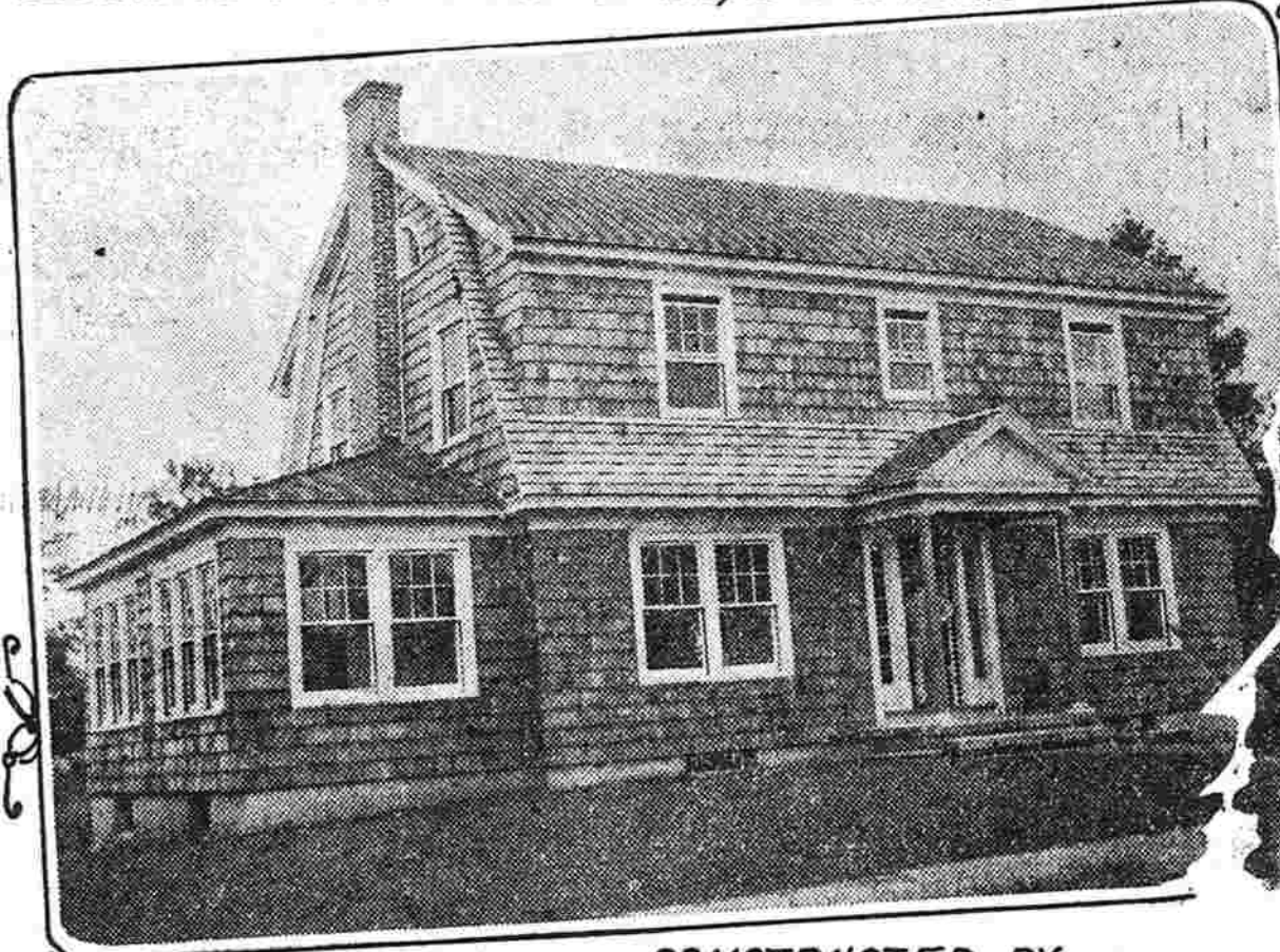
CONSTRUCTED BY GUSTAVE SCHREIBER AND SONS - SCARBOROUGH RD.
